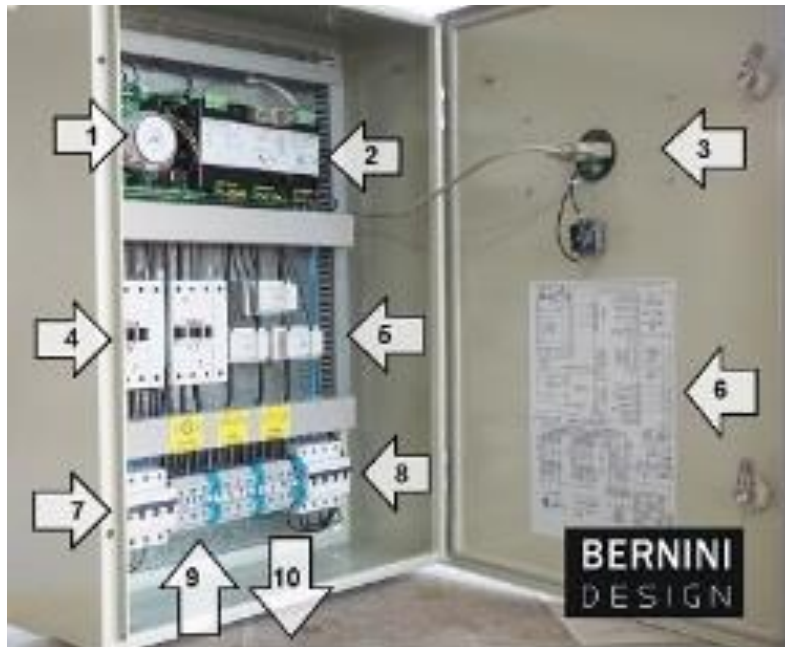
[1] BATTERY CHARGER [2] INTERFACE BOARD [3] AUTOMATIC TRANSFER SWITCH CONTROLLER [4] CONTACTORS [5] CURRENT TRANSFORMERS [6] CABINET DOOR [7] [8] CIRCUIT BREAKERS [9] [10] TERMINAL BLOCKS
